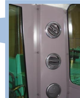
Column integrated ventilation hole for effective air conditioning
